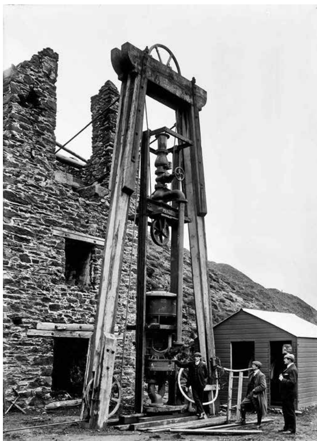
Taylor's shaft at Tywarnhayle c1907. The newly installed electric pumps are seen
